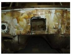
Original positioning of sound deadener under the window wipers. Firewall showing haphazard placement of yellow glue and luckily no signs of rust.
